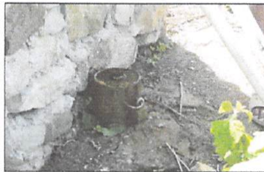
Figure 3. Water overflows in SP.4
